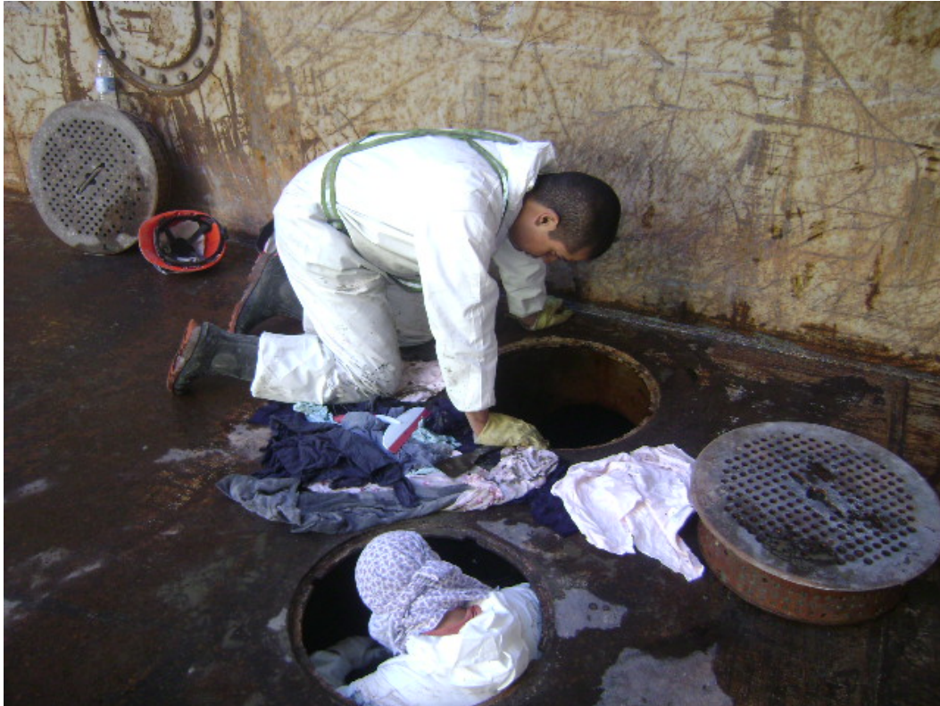
Cleaning Hold Bilge
