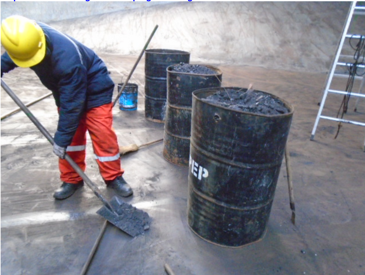
Cleaning and sweeping coal cargo from hold
