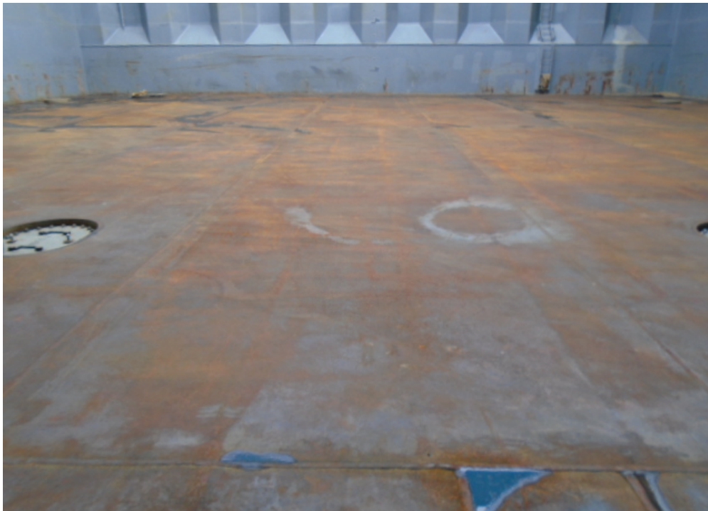
Cargo Hold cleaned ready for “Hold Inspection”
